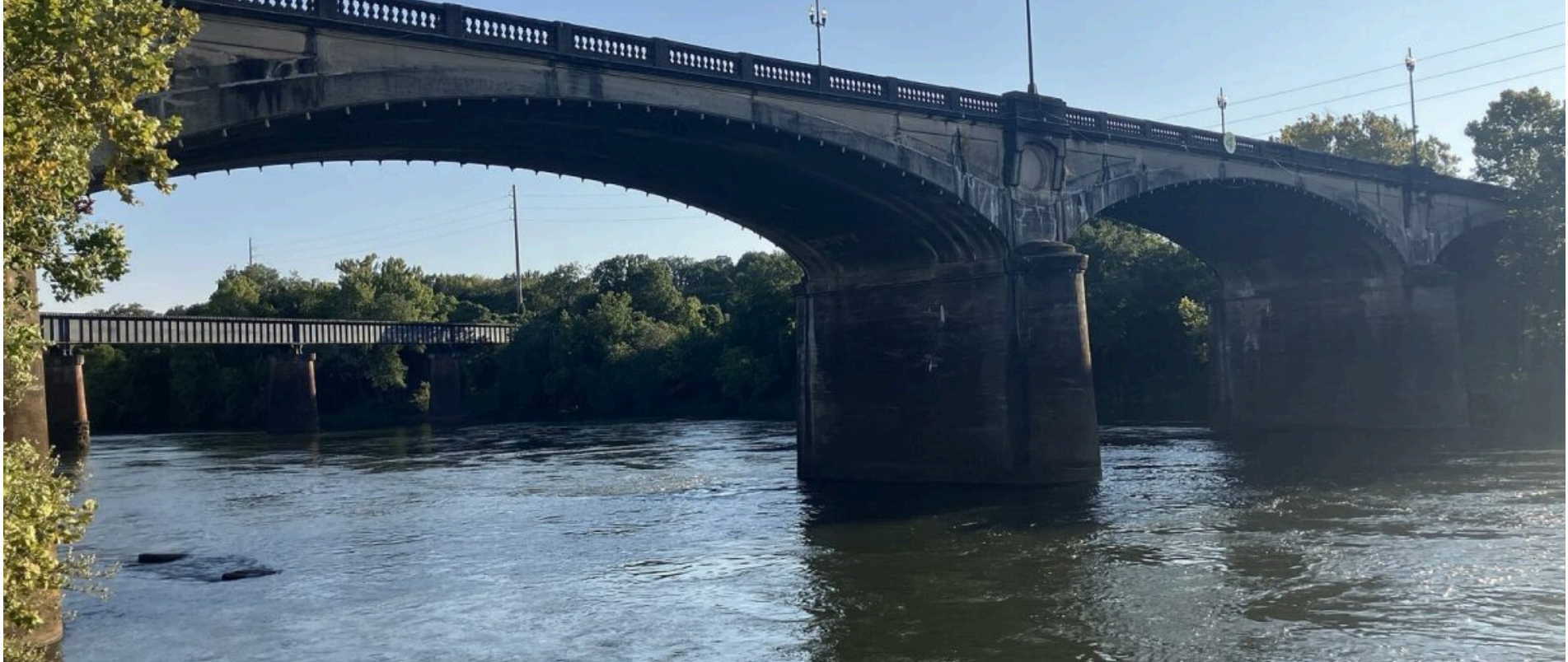
The Dillingham Street Bridge over the Chattahoochee River in Columbus, near the 1865 battle's bridge crossings (file photo). MCCUNICANO / WIKIMEDIA COMMONS (CC BY-SA 4.0)
